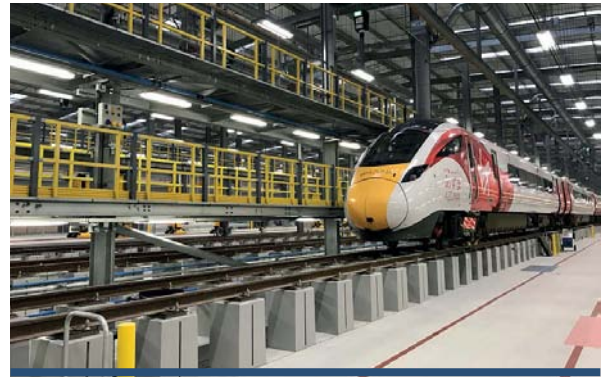
Above GRP open mesh flooring and handrails at Doncaster Carr IEP rail depot 3
